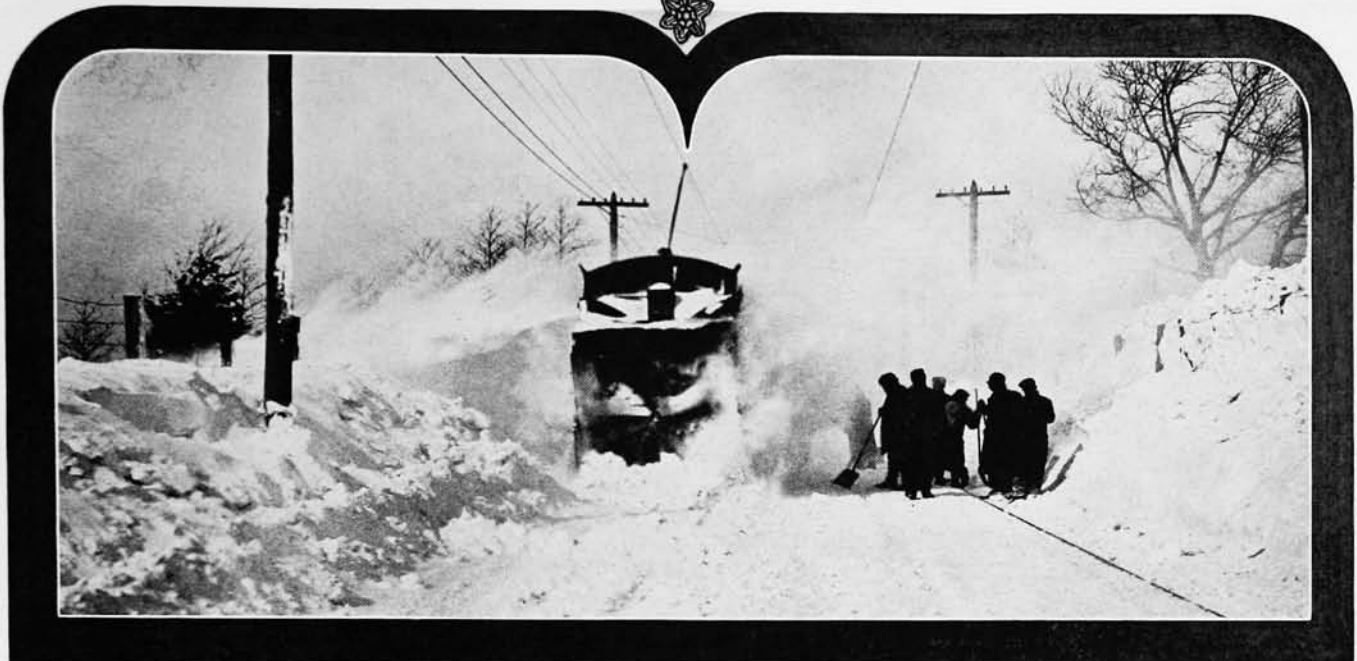
BATTLING A BLIZZARD—1920. Snowplows and emergency storm crew at work clearing the Sea Breeze trolley line.
