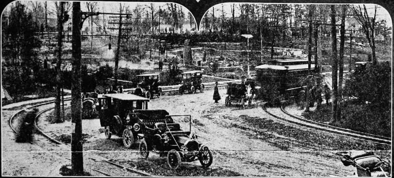
FIRE LEVELS WINDSOR BEACH—1908. View looking east, where St. Paul Boulevard makes right angle turn at lake. Forty cottages (including Unique Social Club) were destroyed, with loss of $125,000.
