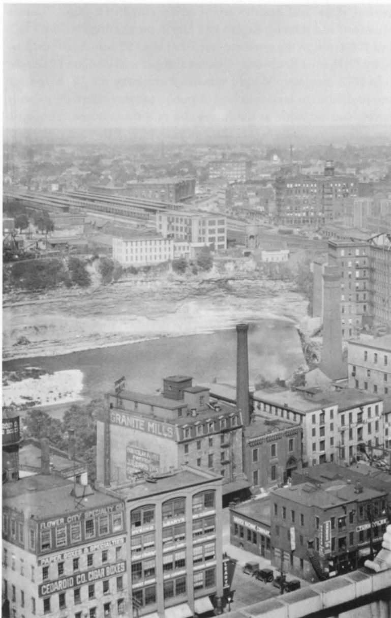
The Granite Mills, Leary's Dyeing Factory are visible in this photograph of the Brown's Race area.
