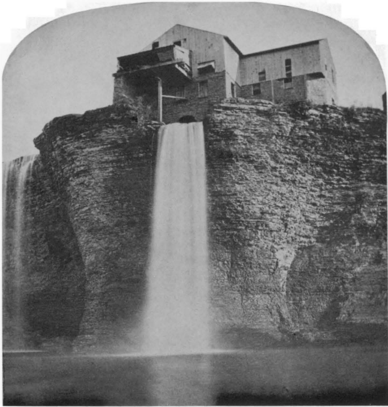
Above: Parson's Saw Mill on Brown's island.
