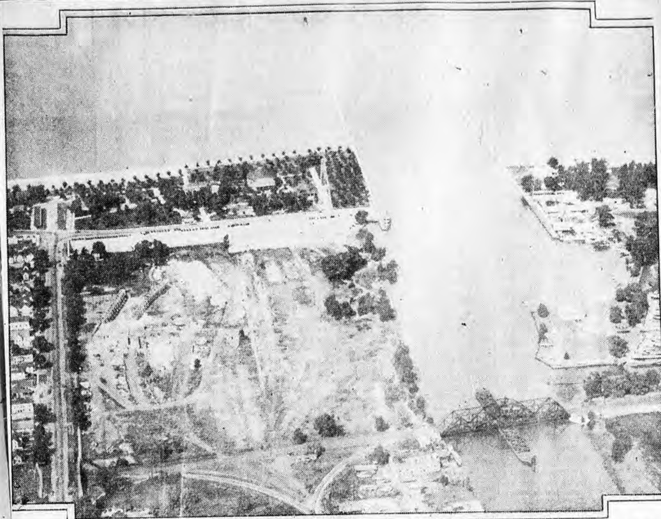
Air view of former blast furnace property on the river front south of Ontario Beach Park taken by Durnherr, Times-Union photographer. The property is shown at the left of the picture. It was announced at the City Council meeting Monday night negotiations had been completed for the purchase of the land by the city from William Bausch for $225,000. The property extends from the beach park to the railroad tracks shown in the extreme lower portion of the picture and from Lake Avenue to the river front. It is sought for the development of Rochester's port facilities.
