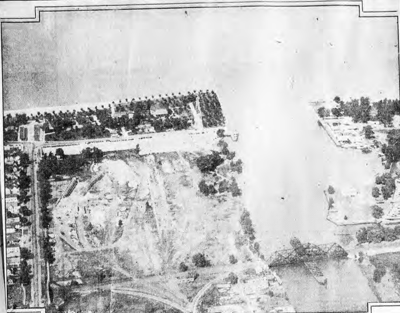
Air view of former blast furnace property on the river front south of Ontario Beach Park taken by Durnherr, Times-Union photographer. The property is shown at the left of the picture. It was announced at the City Council meeting Monday night negotiations had been completed for the purchase of the land by the city from William Bausch for $225,000. The property extends from the beach park to the railroad tracks shown in the extreme lower portion of the picture and from Lake Avenue to the river front. It is sought for the development of Rochester's port facilities.
