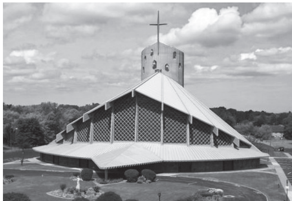
The completed St. John the Evangelist Church, built to serve the expanding population of Greece opened to parishioners in November 1964. Photograph courtesy of William Sauers.
