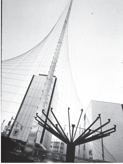
Johnson's original Liberty Pole design, completed in 1965, included a metal tree that served as a fountain in warm months and emitted flames in the winter. From Johnson Slide Collection, Johnson family private collection.
