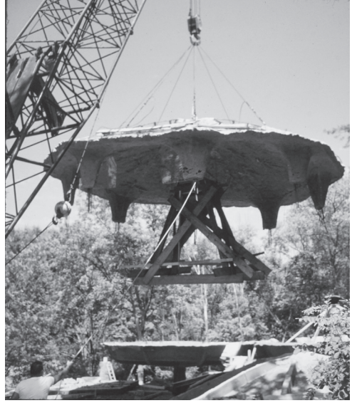
Left: The concrete pods that formed the “Mushroom House” were cast onsite using earth-dug molds. From Johnson Slide Collection, Johnson family private collection. Right: Airlifting a pod into place. From Johnson Slide Collection, Johnson family private collection.
