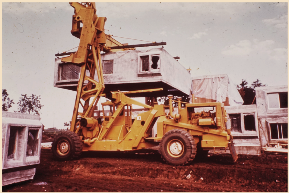
Johnson's Housing Systems company employed his patented portable factory system to build concrete apartment buildings. From Johnson Slide Collection, Johnson family private collection.
