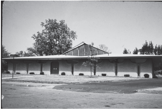
Top: Constructing the concrete wall panels of the Our Lady of Mercy rectory. From Johnson Slide Collection, Johnson family private collection.
