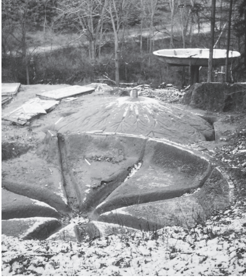
Left: The concrete pods that formed the “Mushroom House” were cast onsite using earth-dug molds. From Johnson Slide Collection, Johnson family private collection. Right: Airlifting a pod into place. From Johnson Slide Collection, Johnson family private collection.
